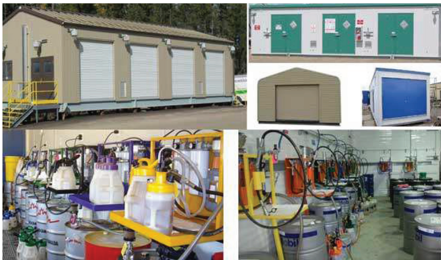
Figure 5. Satellite storage facilities.
